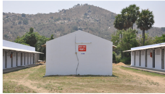
Housing facilities constructed at Foods and Inns. Before, workers were sleeping in houses made of coconut leaves posing a serious fire hazard. Now concrete dormitories have been constructed and fire fighting equipment established
