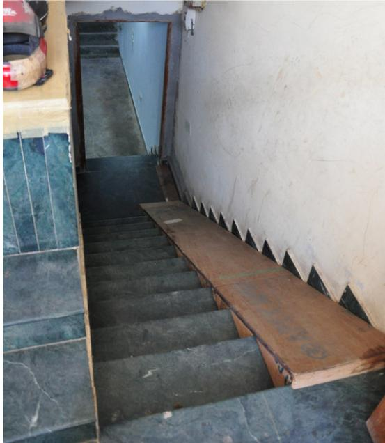
*A slide has been built on the side of the staircase for ease of transportation of heavy bags with leather. Before the workers were carrying the bags on their backs.*
