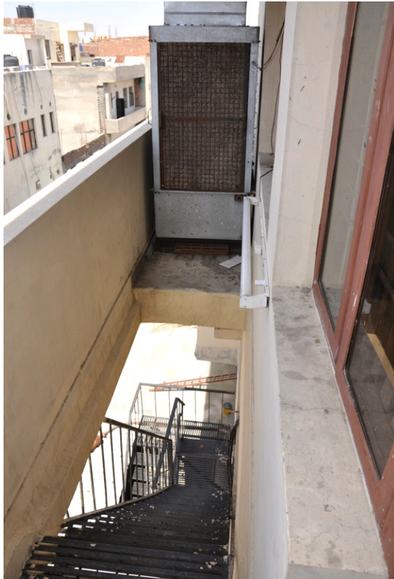
New emergency exit established for quick and safe evacuation. In the background, part of the new air cooling system can be seen
